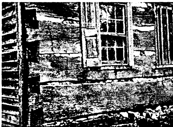
Detail of Structure—Garst House
